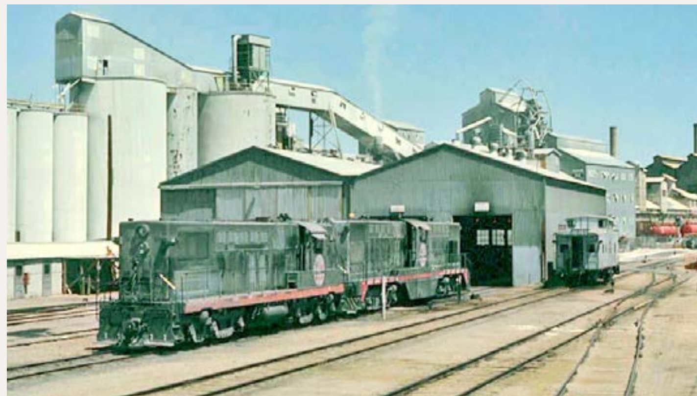
Figure 4: Trona’s Baldwins await their next run in front of the four bay diesel shop. Selective compression can be used to model this structure as a two bay diesel shop on the layout.
