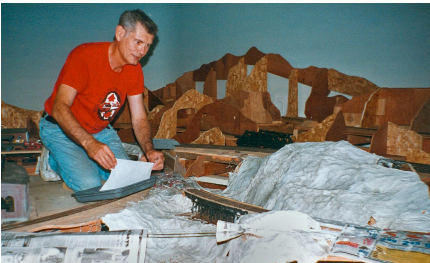
Time for scenery. Bob is dipping paper towels in plaster to make a hard shell scenery base.
