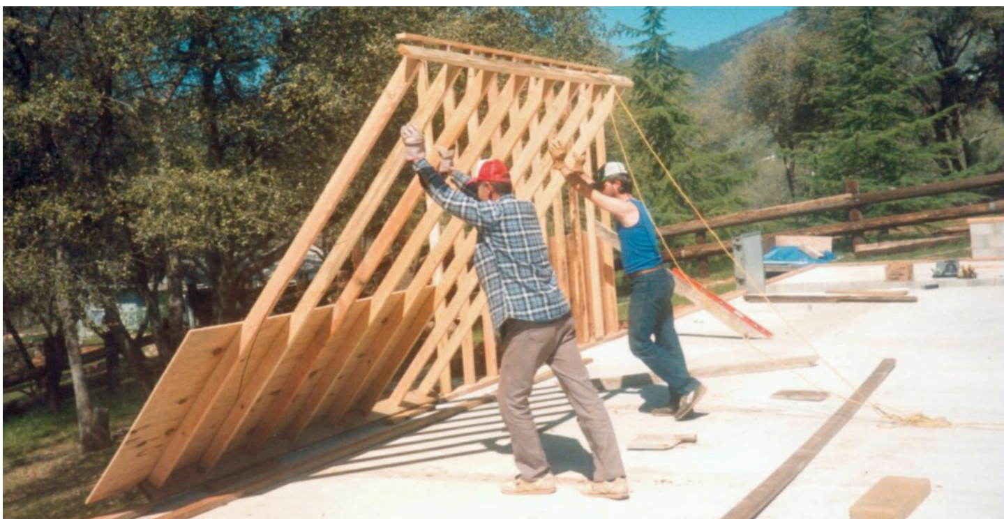
Up go the walls. Bob and son, Tom, are raising the second wall section here.
