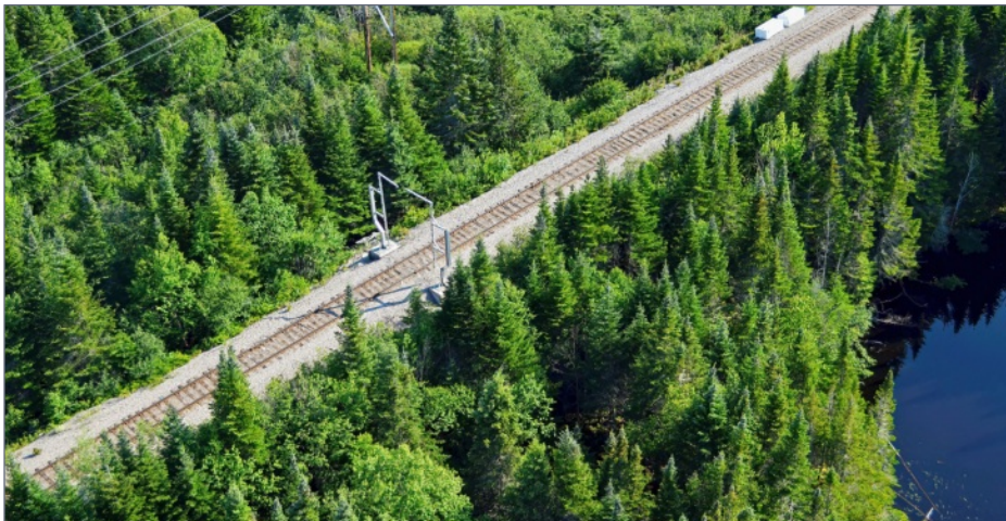
19. A clearance check just north of the bridge ensures that any wide or high loads will be flagged before they get to the bridge. This is another good model to add to the bridge module.
