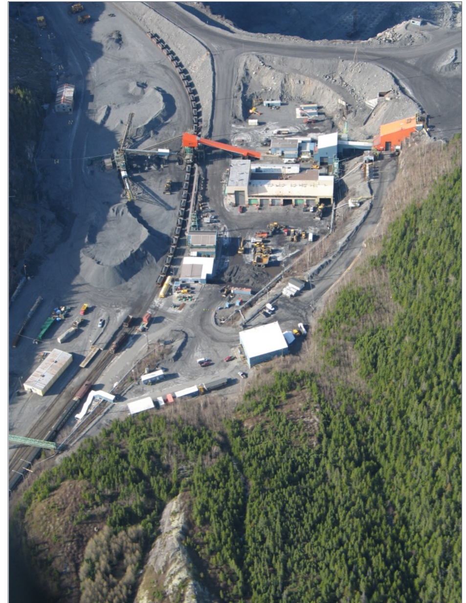
12. An overview of the mine loadout and facilities at the open pit. A loaded ore train and a lone RS-18 give scale.
