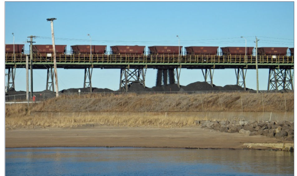
15. Dumping ore cars at the Havre St. Pierre ore dock for loading onto a conveyor.
