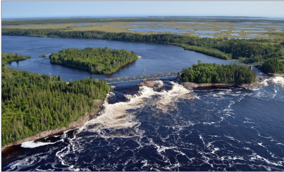
18. The QIT bridge over the Romaine River just northwest of the airport begs to be modeled on one of the later phases of the TOMA layout.
