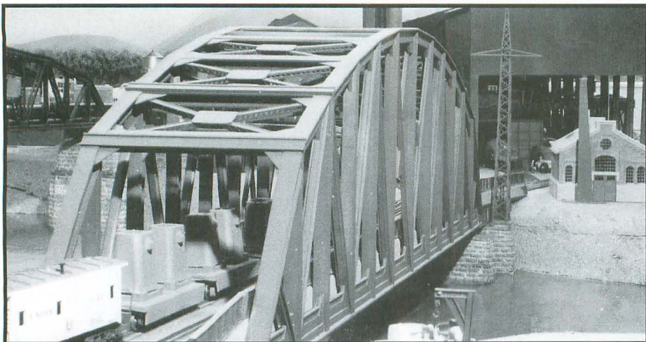
PHOTO 15. The Union RR "Hot Metal Bridge" at Rankin, Pennsylvania just across the Monongahela River from Homestead. This unusual bridge has solid steel flooring, and concrete and girder walls to prevent bridge damage and possible explosions from hot metal spills. Here, a URR switcher shoves a string of ingots onto the bridge, coming from Homestead Works, followed by a yellow URR caboose.
