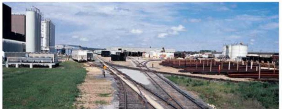
FIG. 2 PROTOTYPE PARK. Progressive Rail's Airlake Industrial Park is a compact complex of tracks and transfer points that serve a wide variety of industries. Jim Hediger photo
