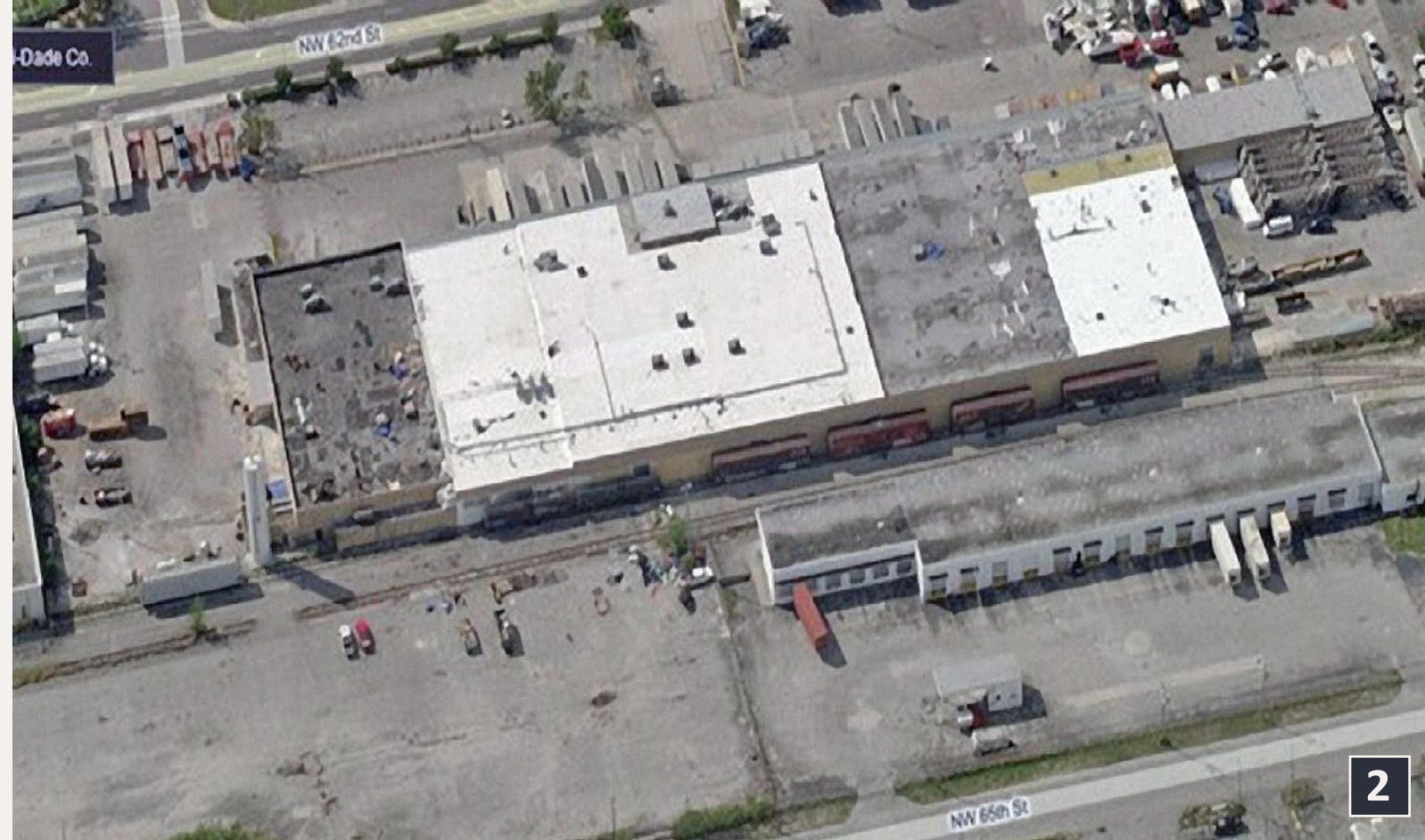
2: From the air, it's easy to see how the various car spots and sorting tracks line up alongside a commercial bakery served by the Florida East Coast railroad in Miami. (Aerial view facing due south.)
