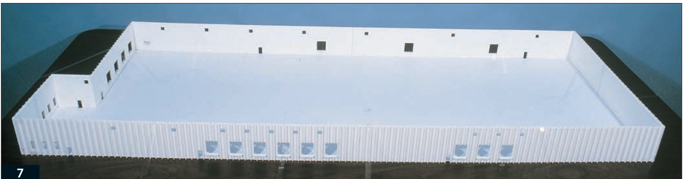
7 The walls are temporarily positioned around the warehouse subfloor so the locations of the ground-level doors can be marked.
