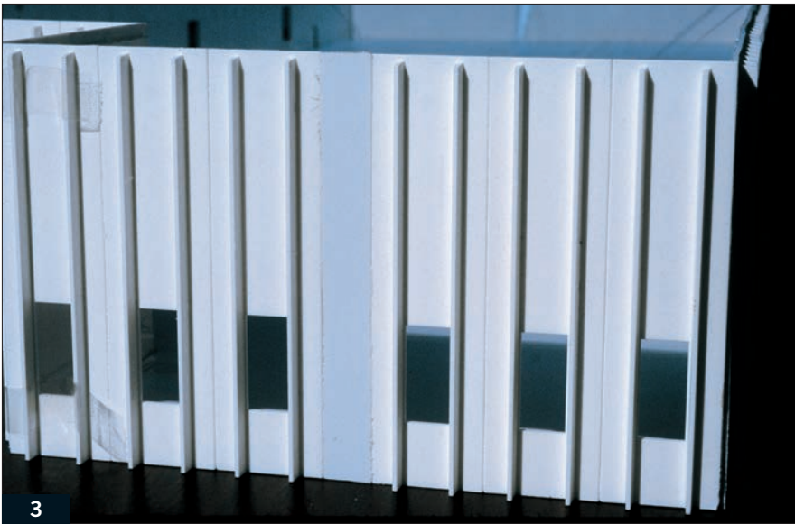
3 You can see windows attached between the ribs in the paneling, and the gray strip in the center is the spacer added between panels. This allowed me to customize the dimensions of the warehouse.
