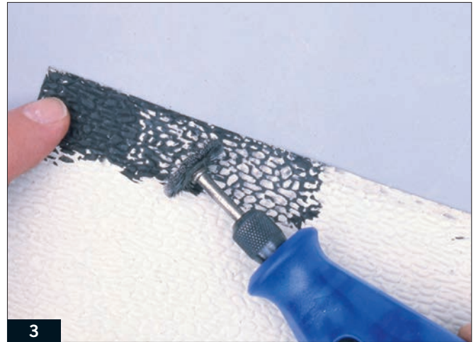
3 A motor tool with wire brush removes most of the black paint from the surface of the fieldstone sheet, leaving what appear to be black shadows in the recesses between the rocks.
