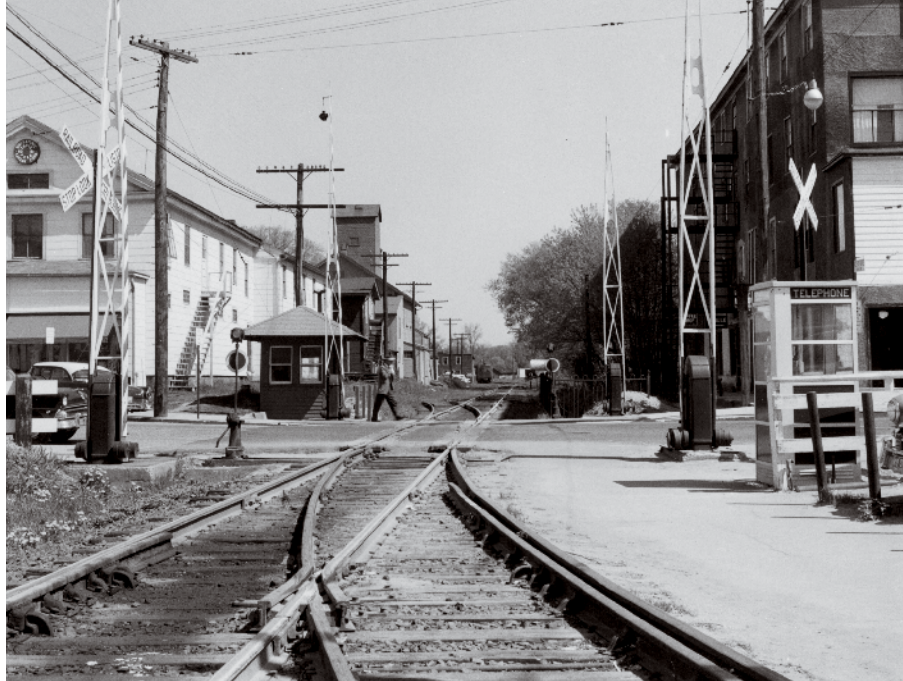
Fig. 1 Prototype grade crossing. Grade crossings have changed since Douglas Smith took this photo in 1958. Note the paved crossing with timbers on each side of the rails, the manual gates, and the crossing shanty.
