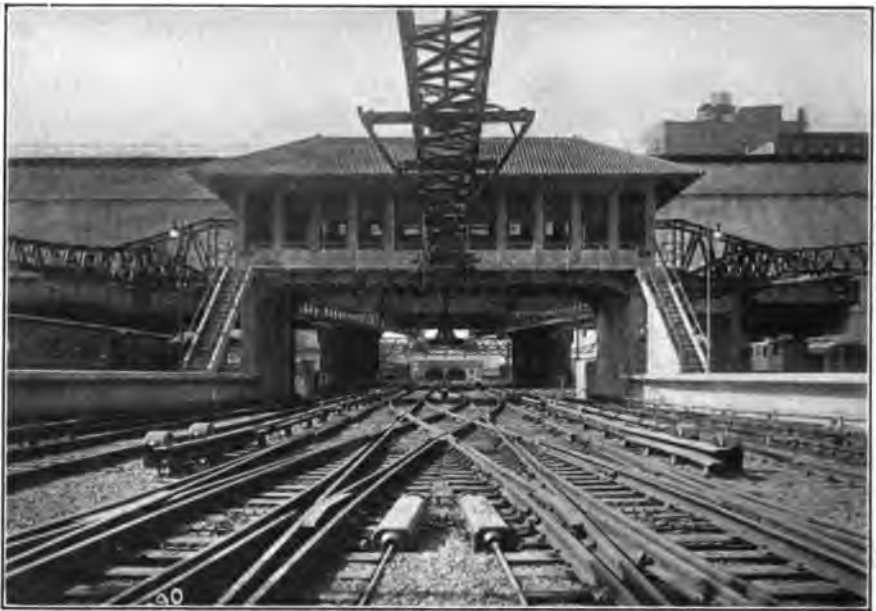
FIG. 24.—Tower "A," Pennsylvania Station, New York.
