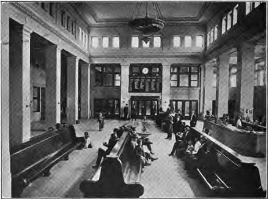
FIG. 137.—Train indicators in Illinois Central Station, Memphis.
