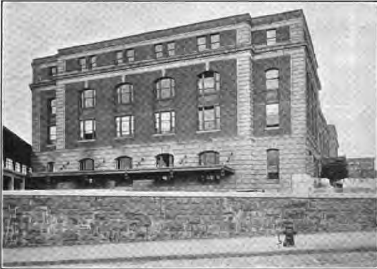
FIG. 51.—Exterior of Rochester Station.
