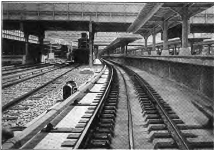
FIG. 18.—View in Grand Central Station, showing track construction, raised platform and train sheds.
