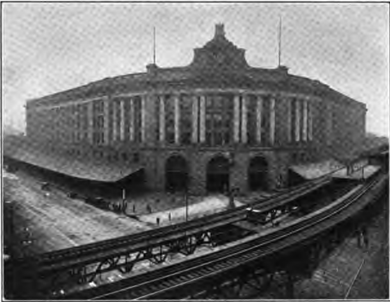
FIG. 73.—South Station, Boston.
