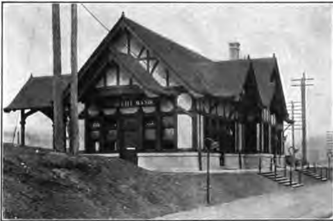
FIG. 162.—Concrete and stucco station, New York Central.
