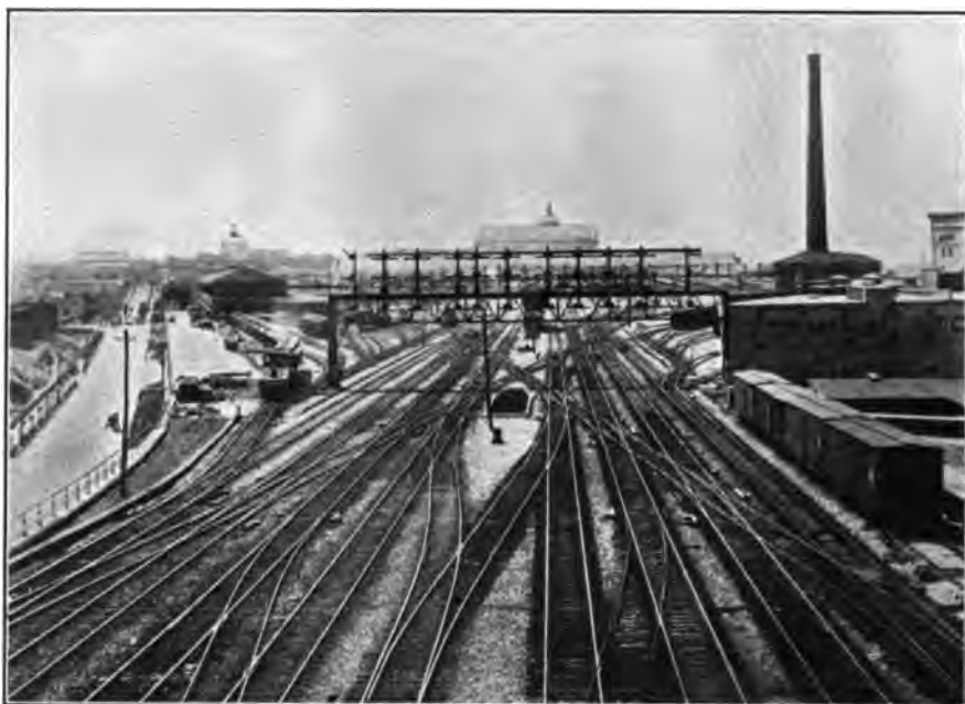
FIG. 36.—Approach tracks to Union Station, Washington. Parallel and alternative routes are provided.
