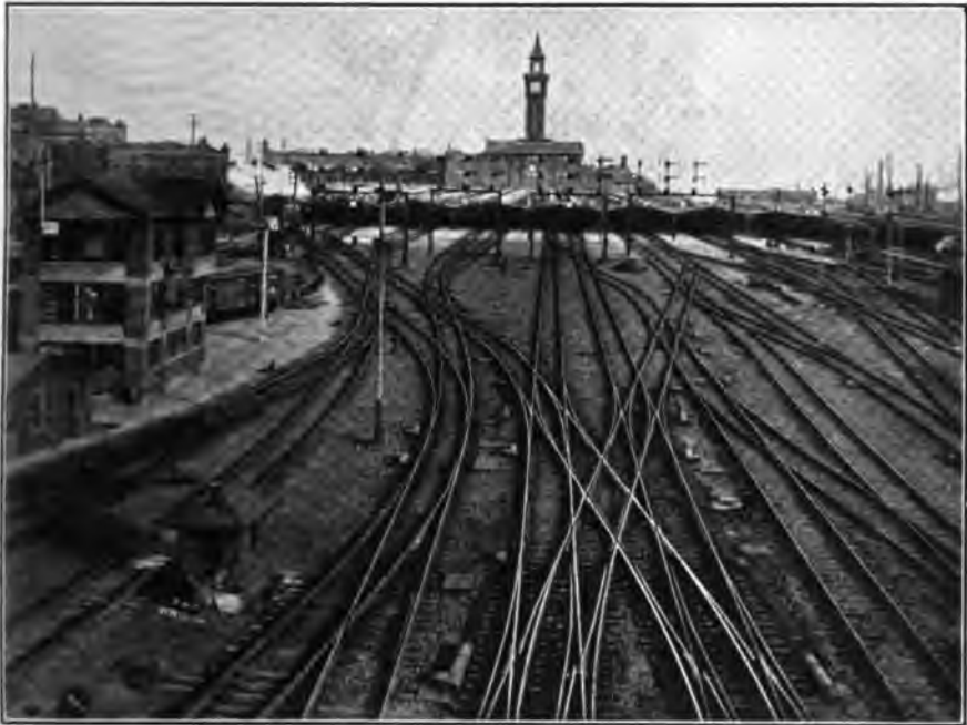
FIG. 28.—Interlocking at Lackawanna Terminal, Hoboken, N. J.
