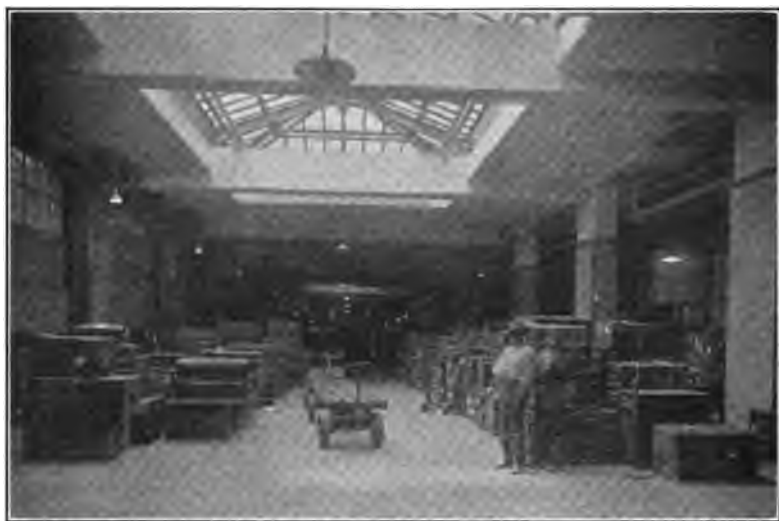
FIG. 141.—Baggage room, Grand Central Terminal, New York.
