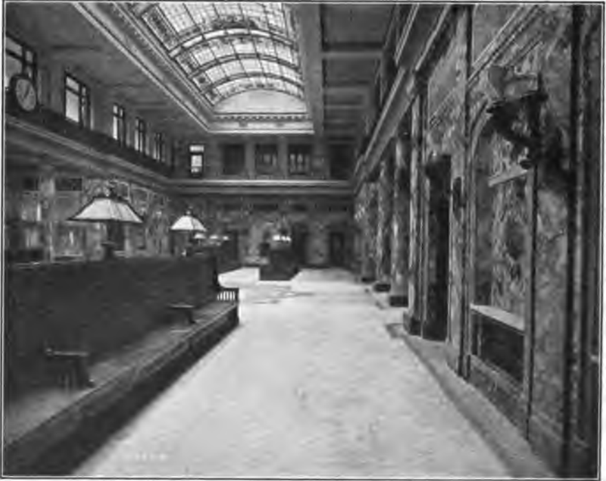
FIG. 44.—Waiting room of Scranton Station.
