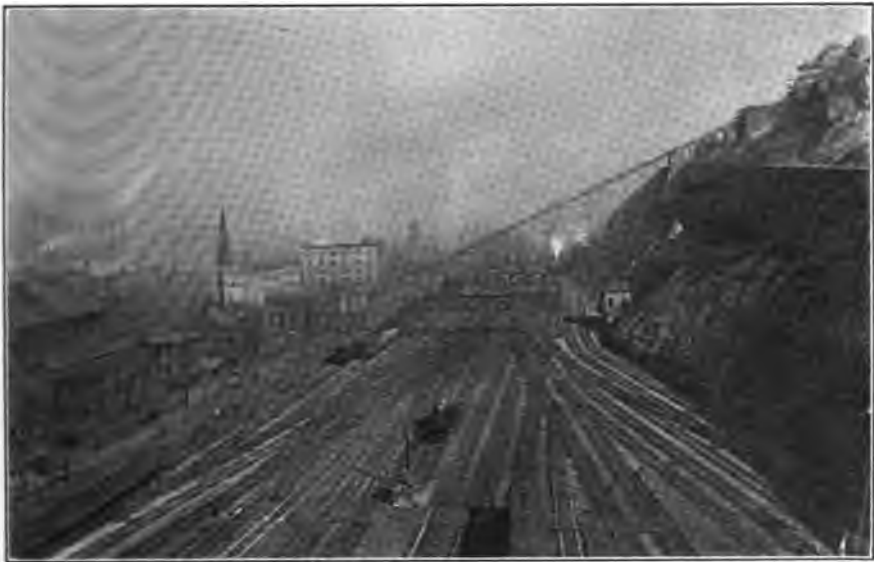
FIG. 37.—Looking eastward from Pennsylvania Railroad Terminal, Pittsburgh. There is double line of crossover tracks running in both directions from right to left and from left to right, providing facilities for parallel and alternative movements in either direction.
