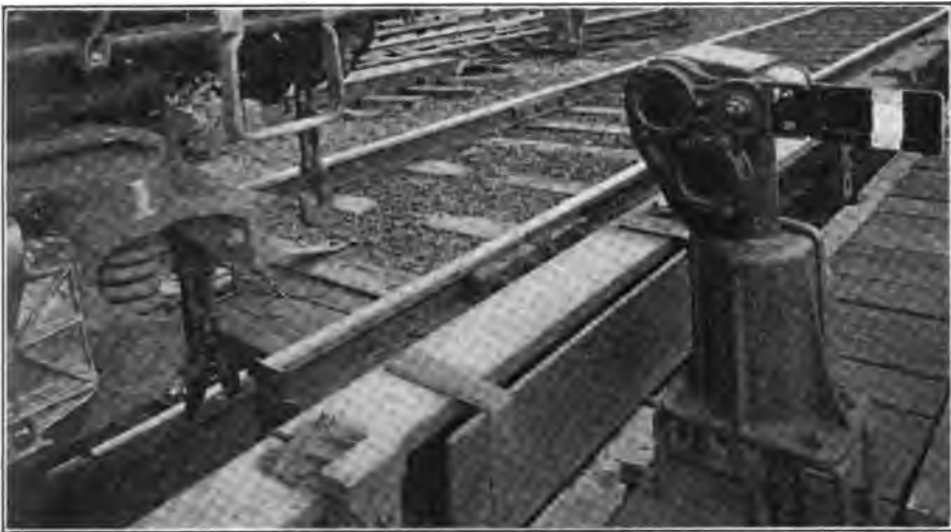
FIG. 207.—Automatic stop on the Interborough Rapid transit.
