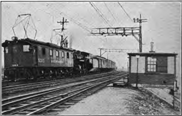
FIG. 195.—Hoosac tunnel electrification, Boston & Maine.
