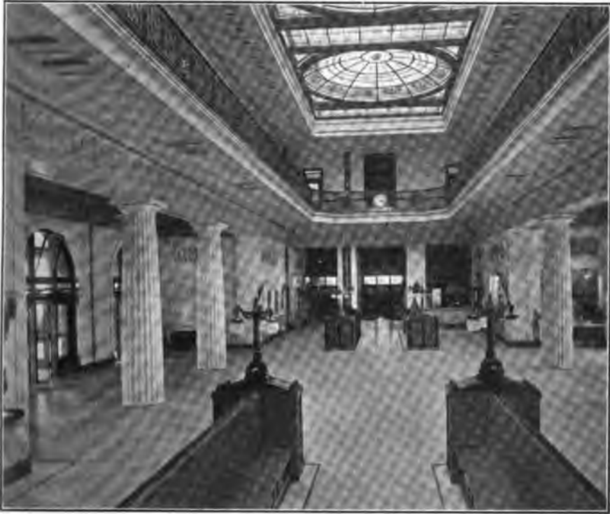
FIG. 64.—Waiting room of Baltimore Station.
