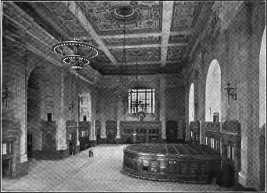
FIG. 62.—Ticket lobby of Kansas City Station.
