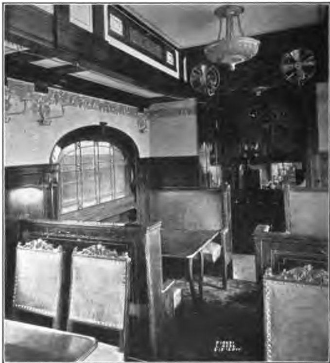
FIG. 217.—Serving counter of New Haven dining car, showing small space available.
