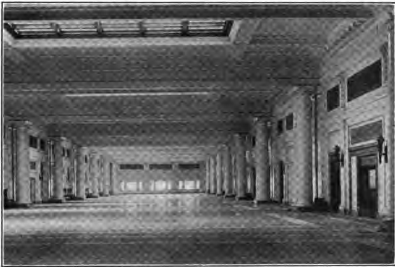
FIG. 106.—Upper ferry concourse of Lackawanna Station.
