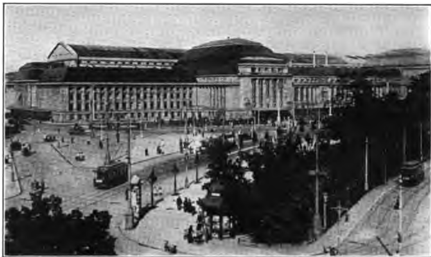
FIG. 173.—Station in Leipsic, Germany, the largest in Europe.
