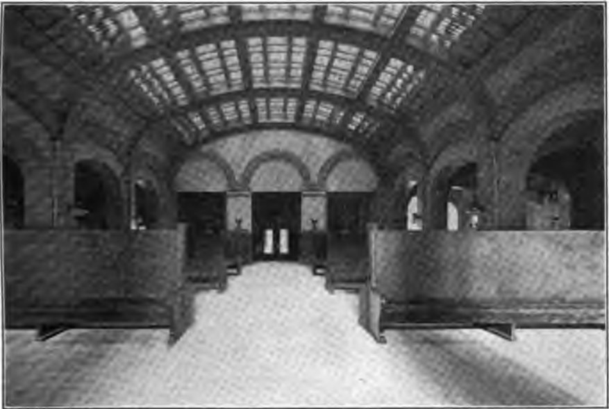
FIG. 55.—Winnipeg Station waiting room.
