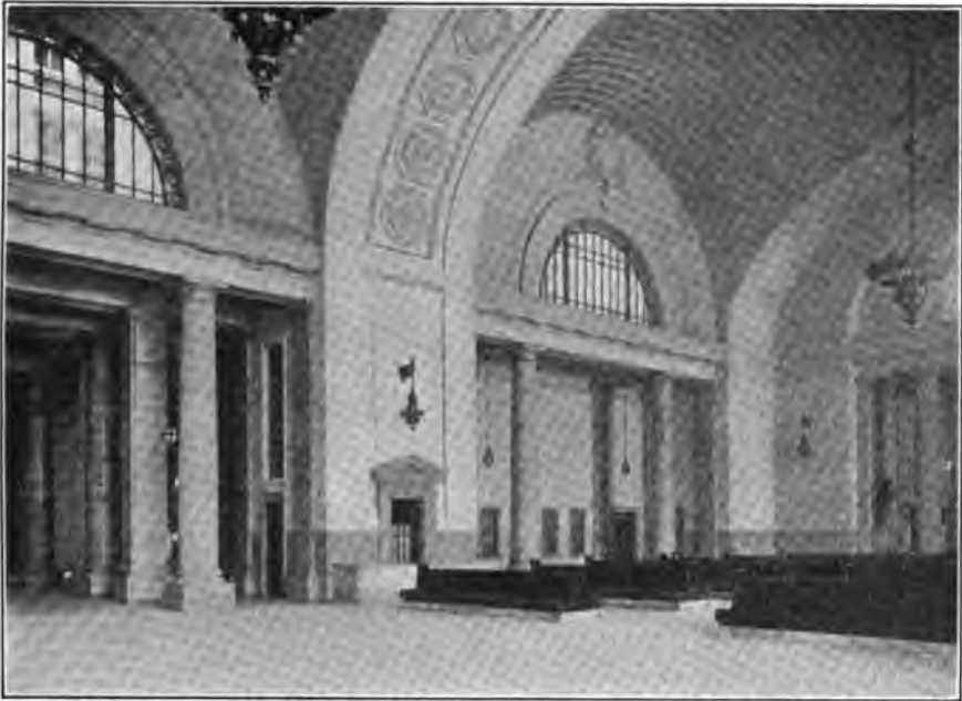
FIG. 48.—Waiting room of Detroit Station.
