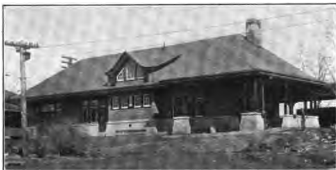
FIG. 156.—Concrete and wood station, New York Central.
