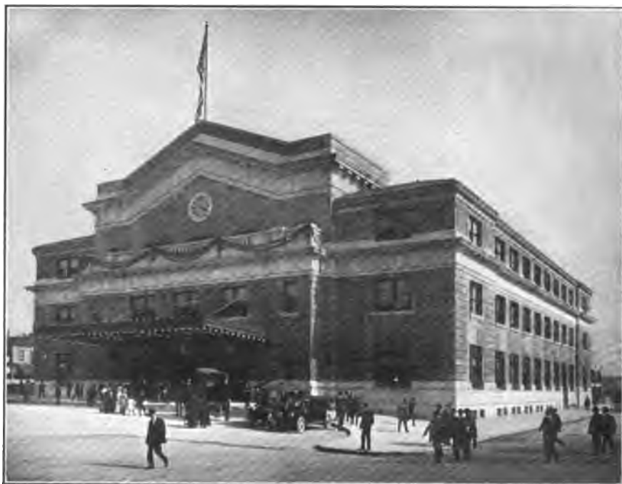
FIG. 84.—Exterior of Oregon-Washington Station, Seattle
