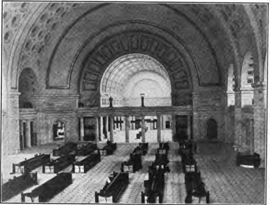
FIG. 78.—Waiting room of Washington Station.
