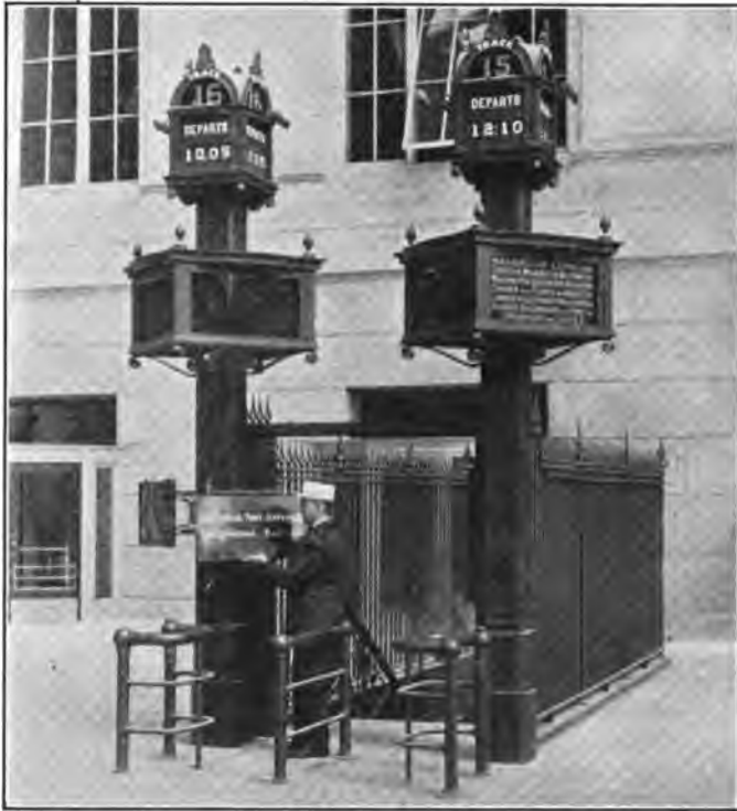
FIG. 134.—Method of adjusting indicators shown in Fig. 133.
