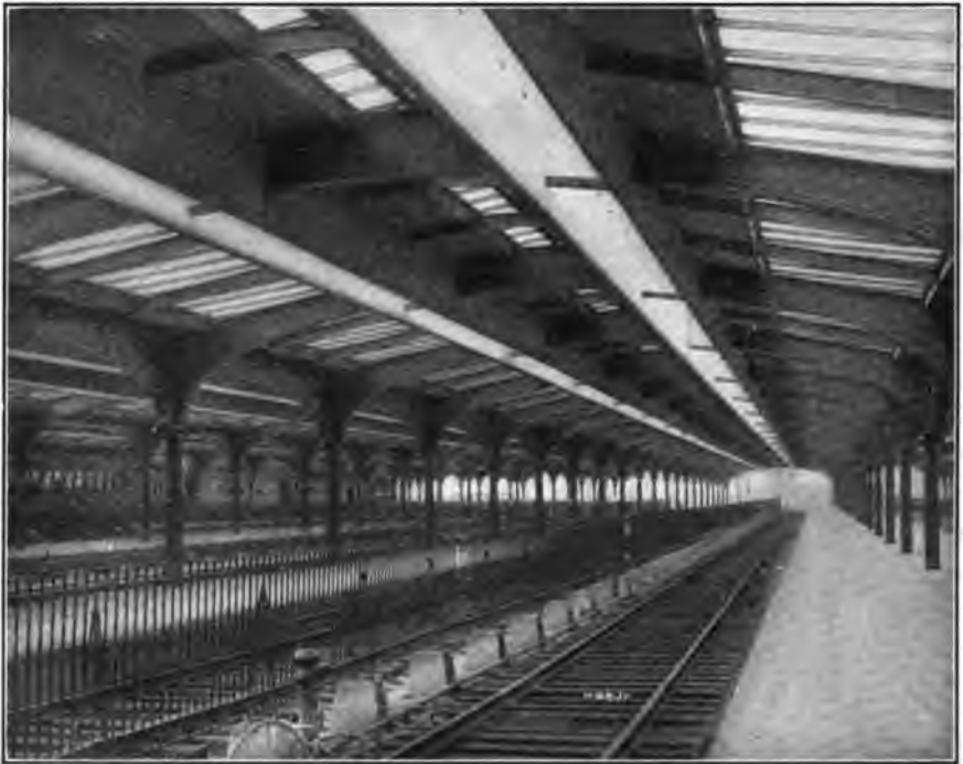
FIG. 20.—Bush train shed at Hoboken—the first of its kind.
