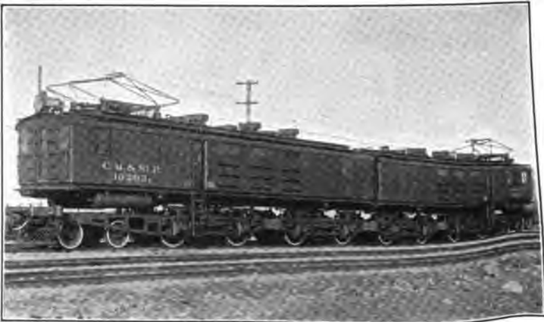
FIG. 188.—Locomotive used on St. Paul's electrified line.
