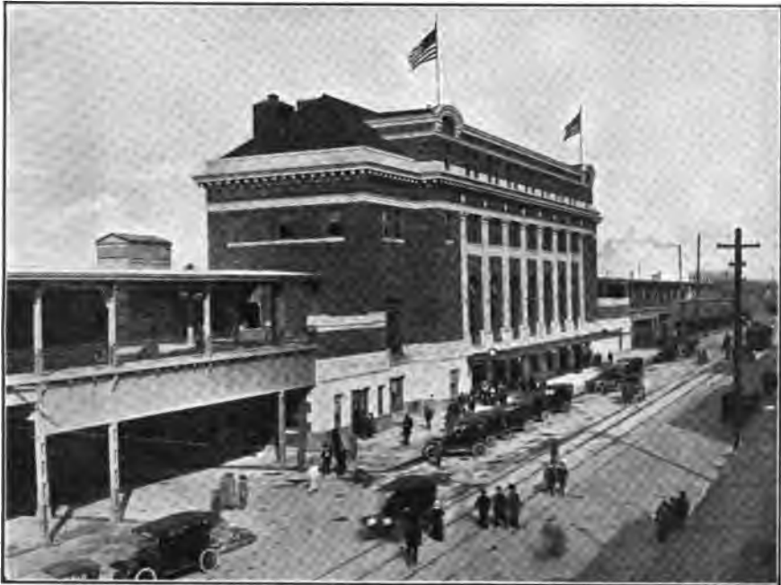
FIG. 57.—Exterior of Spokane Station.
