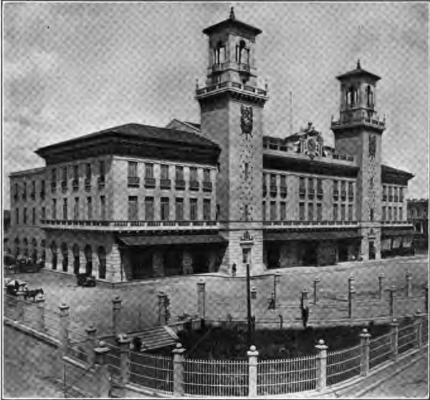
FIG. 184.—Central Station, Havana.
