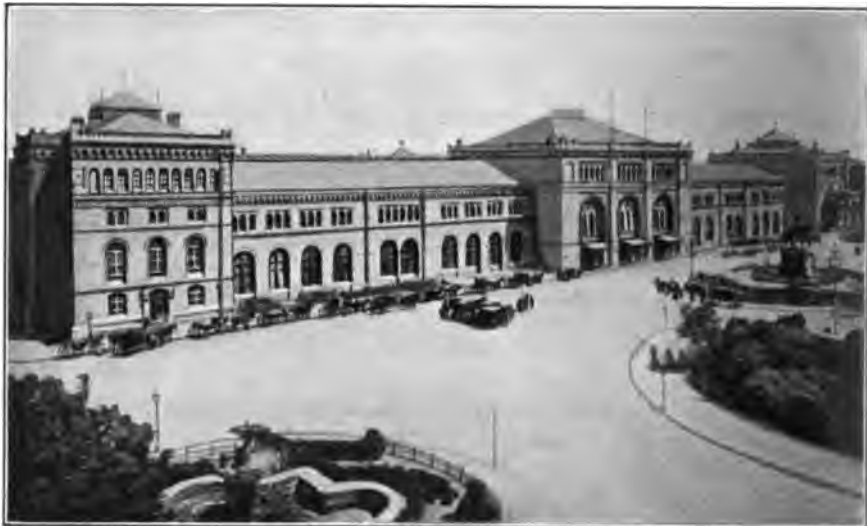
FIG. 174.—Station in Hanover, Germany. 1
