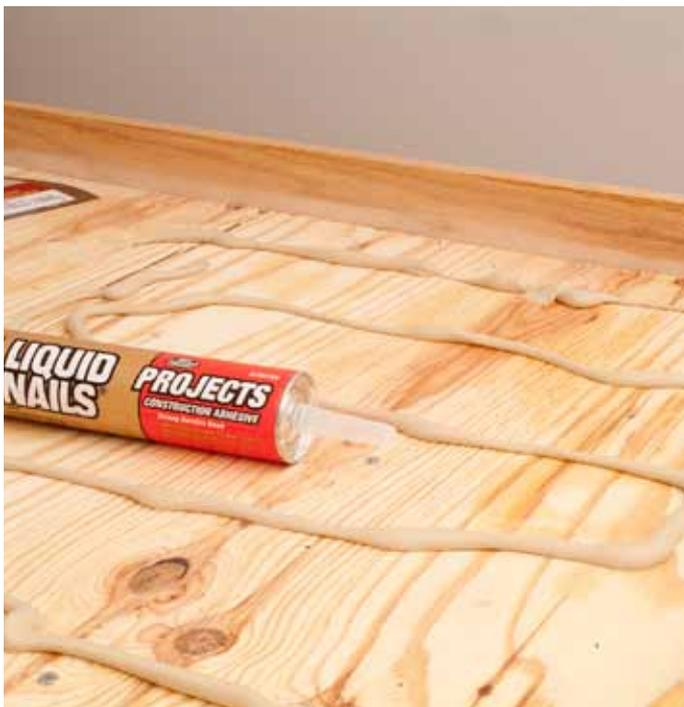
We used Liquid Nails For Projects brand latex adhesive ([www.liquidnails.com](http://www.liquidnails.com)) to bond the foam to the plywood. Bonding the foam to the plywood gives the plywood a little more strength. If you find that the foam wants to lift off of the plywood, use dry-wall screws to hold it in place while the Liquid Nails dries. You may remove the screws later.
