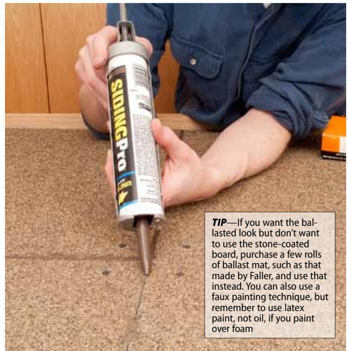
After the Liquid Nails dried, we used brown acrylic caulk to hide any seams and fill any gaps between the foam boards. Once our foam-covered framework was done, we had a tabletop that already looked realistic, if a bit barren. At this point, the surface was ready for us to install track, which we'll cover next in our Build a Retro Railroad instructions.
