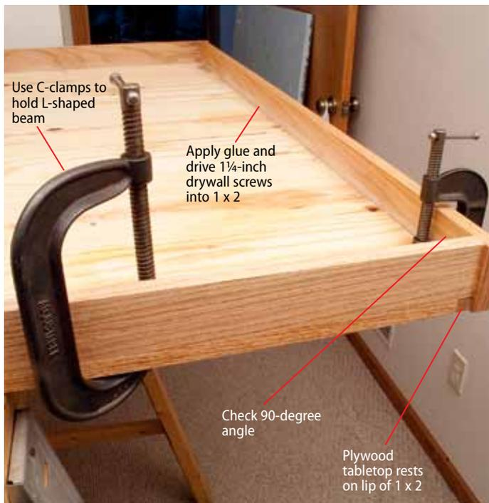
After allowing the glue to dry, we installed the L-shaped beams along the plywood edges. We used clamps to temporarily secure the 1 x 2 lip of an 8-foot beam to the underside of the plywood. We confirmed that the 1 x 3 fit at a right angle to the tabletop and then used wood glue and drywall screws to attach the beam.
