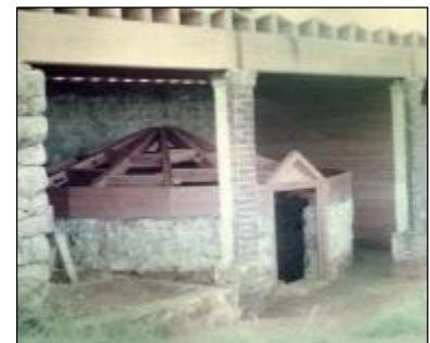
Thomas Jefferson's ice house at Monticello (roof under reconstruction in the 1950s)
