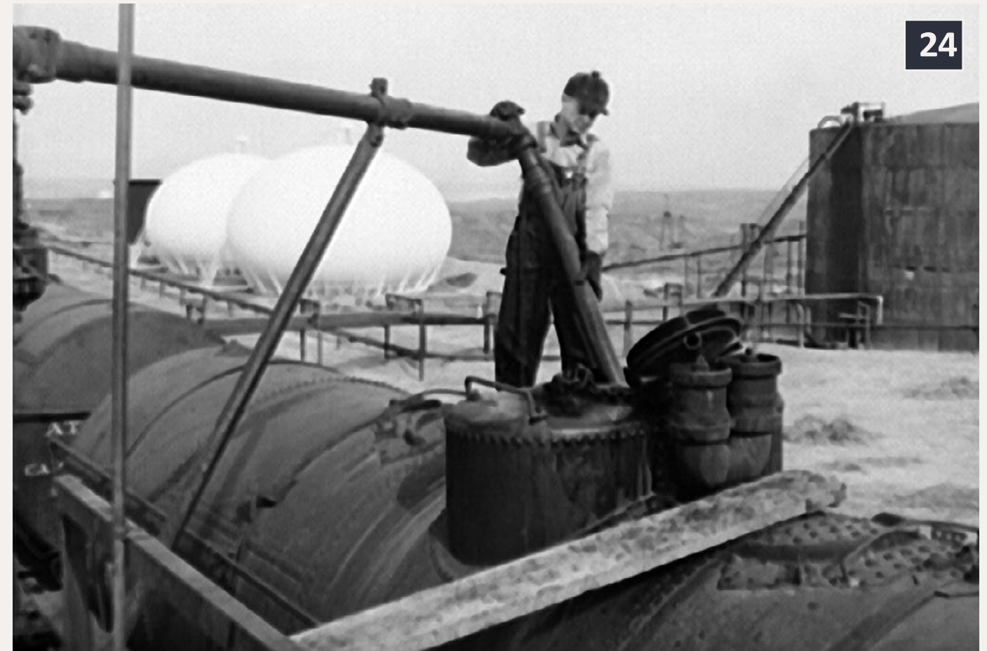
24: Loading oil at the Phillips refinery in Borger, Texas in November 1942. The boom with rotating pipe joints is fed from the platform. The workman has crossed to the tank from the platform at left with a length of lumber. – John Vachon photo, Library of Congress, no. LC-USW3-011638.
