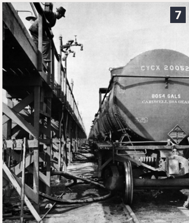
7: Tank car unloading hoses at Standard Oil's plant in Bayway, New Jersey. The platform above is for car loading. –Standard Oil Company photo, Rob Evans collection.
