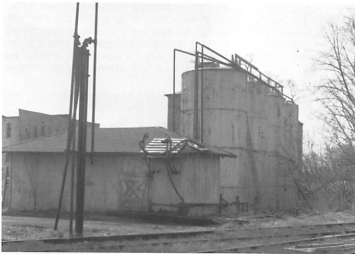
The plant at Pecatonica, Ill., (next to the now-abandoned C&NW) featured an unusual header (compare to the "standard" type modeled in this feature) and a collection of vertical storage tanks. The simple wooden building serves as the pumphouse, truck loading rack and warehouse in one package.
