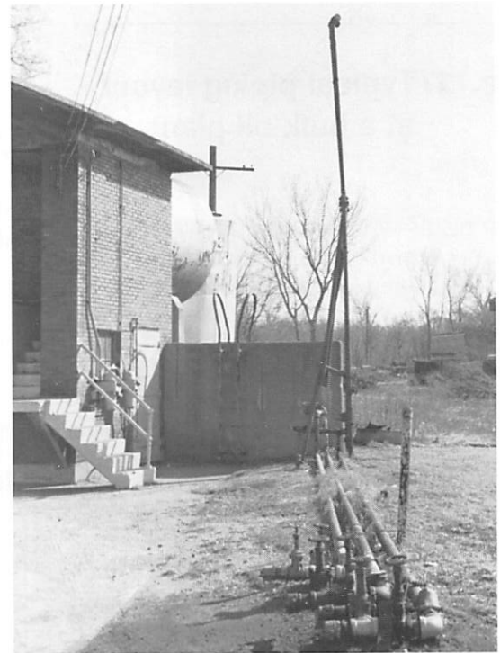
Two views of a typical header used for unloading tank cars. Above: The tall unloading pipes swiveled down to the right, over tank cars, and another pipe attached at the elbow reached through the dome to pump out the petroleum products. Left: This view clearly shows the two unloading pipes that are used to keep separate high and low flash fuels.
