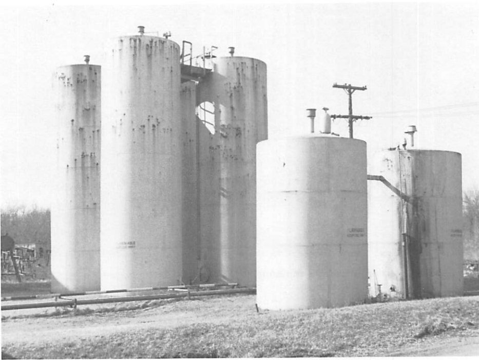
Left: Bulk oil plants all feature their own distinctive collection of oil tanks. This plant in Freeport, Ill., has only vertical tanks, of varying sizes. Note the piping on the ground which is "color-coded" to signify the type of fuel carried. Below: A close-up look at the piping at the base of a header.
