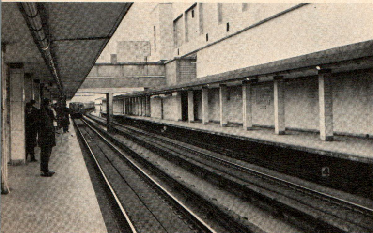
BELOW: Davisville Station on Toronto's new rapid transit system is in open cut. Roadbed is unique; is built to provide fast draining.
