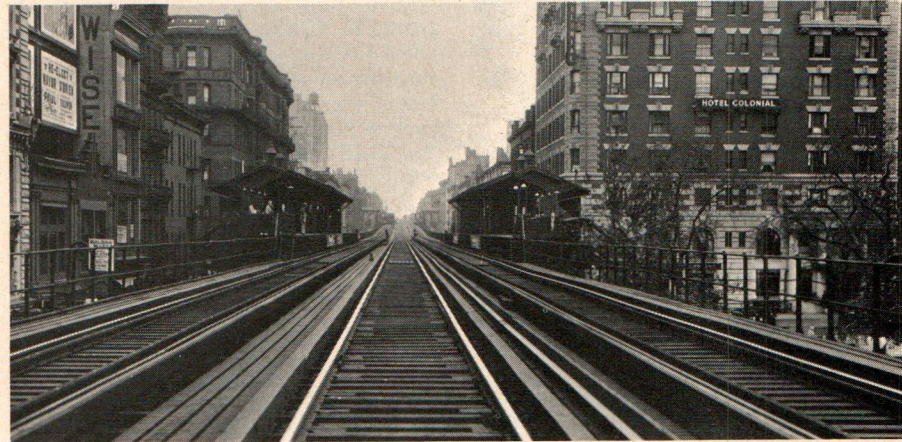
ABOVE: New York's 9th Ave. El in 1872, two years after conversion from cable operation. Space saving el structure was early design.
