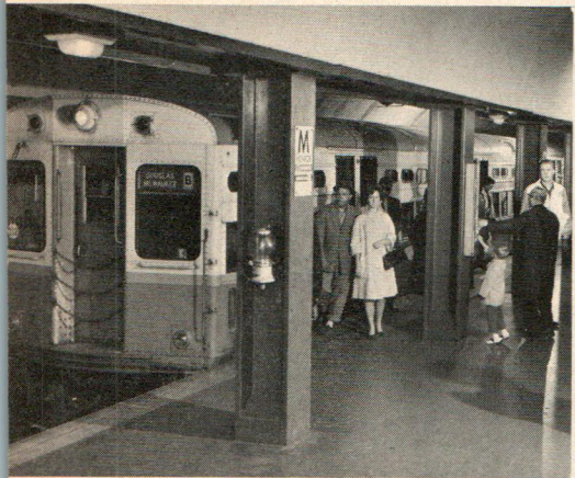
Chicago's loop is surrounded by el structure with white columns and grey superstructure. CTA el cars are converted from PCC parts.
