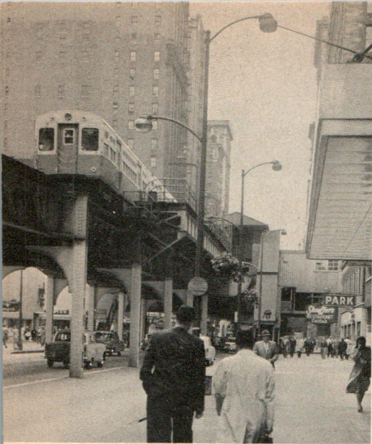
Chicago's loop is surrounded by el structure with white columns and grey superstructure. CTA el cars are converted from PCC parts.
