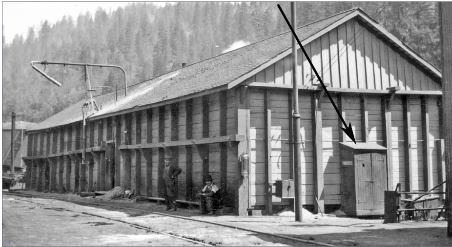
23. The south end of the SP sand house at Dunsmuir had a fire equipment cabinet, indicated by the arrow, and it was painted bright red. Notice it is supported off the ground. This is the type of cabinet I decided to model. SP photo, Shasta Division Archives, courtesy Bob Church
