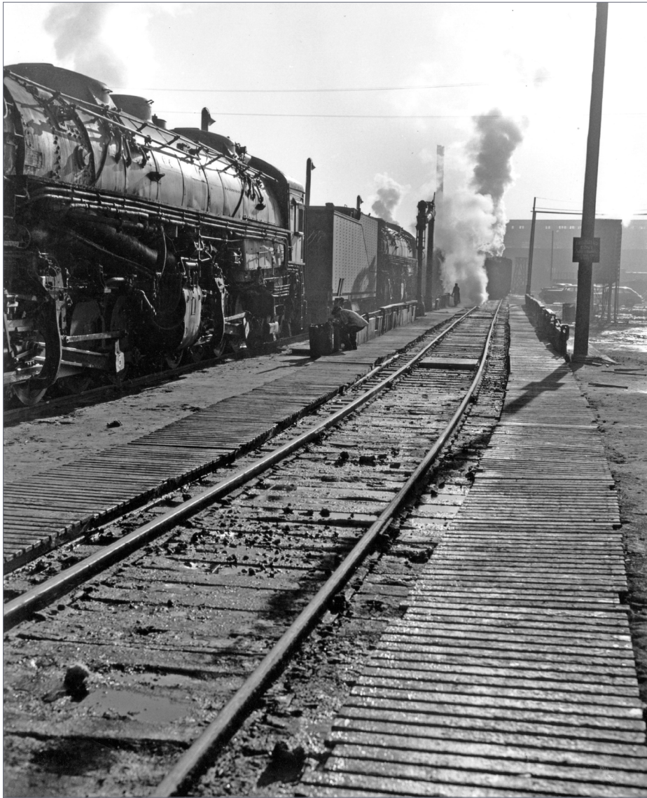
5. This photo of the wash rack north of the roundhouse at SP's Taylor Yard in Los Angeles, taken in the summer of 1950, shows the duckboards provided so workmen's feet could mostly stay out of the accumulated oil and water in the area. Richard Steinheimer photo, DeGolyer Library
