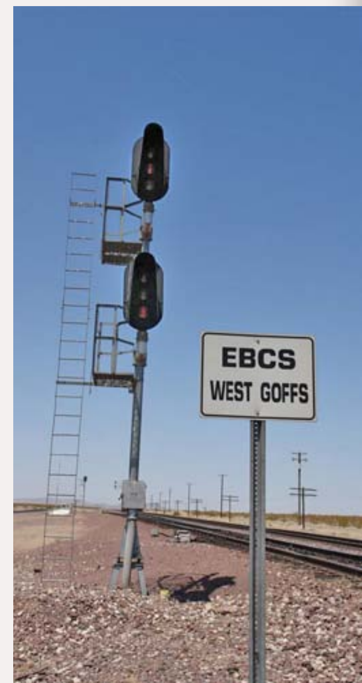
Figure 7. Eastbound signal mast.
