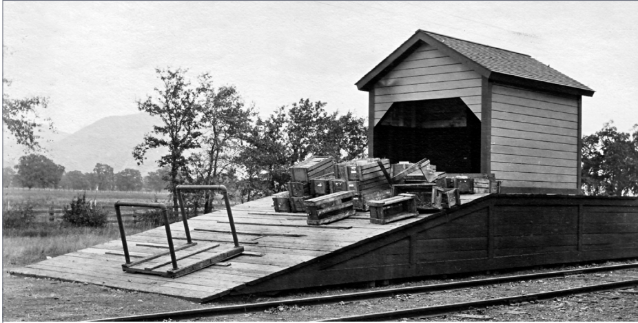
8. The freight shelter at Los Guilicos, California, north of Kenwood on the Santa Rosa Branch, in a 1912 photo from Bender's book. This 10 x 12-foot shed stood on a 16 x 20-foot platform, not counting the ramp. SP photo, Shasta Division Archives
