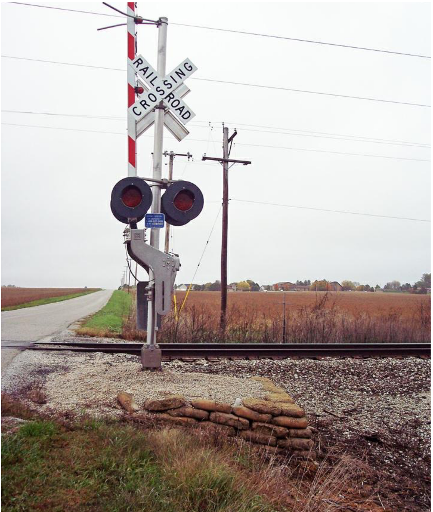
These two photos show how the Toledo Peoria and Western made some retaining walls in Illinois with sacks of concrete mix. You can tell by the shape that the bags were stacked up dry, and when it rained, the concrete set.
