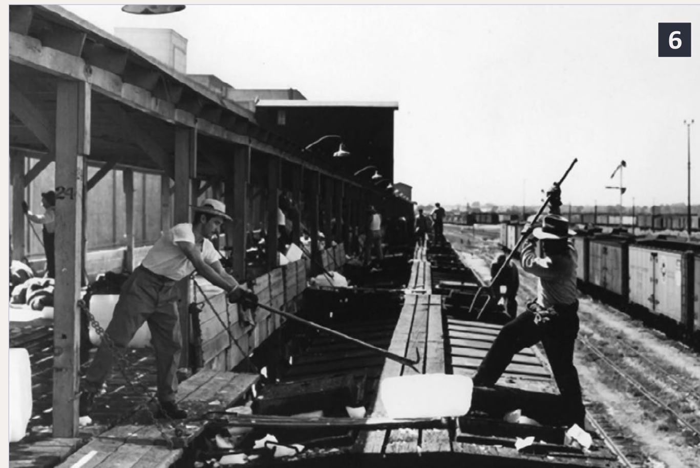
6: This superb photo by Jim Morley at Roseville shows men actively handling ice. The 300-pound blocks on the deck are being split into quarters. The man on the apron is called the “passer,” and he uses a pickaroon to move quarter blocks over a bridge, to the man working at the hatch. With the bident, the “chopper” at the hatch chops the ice to the needed size. – Author’s collection.
