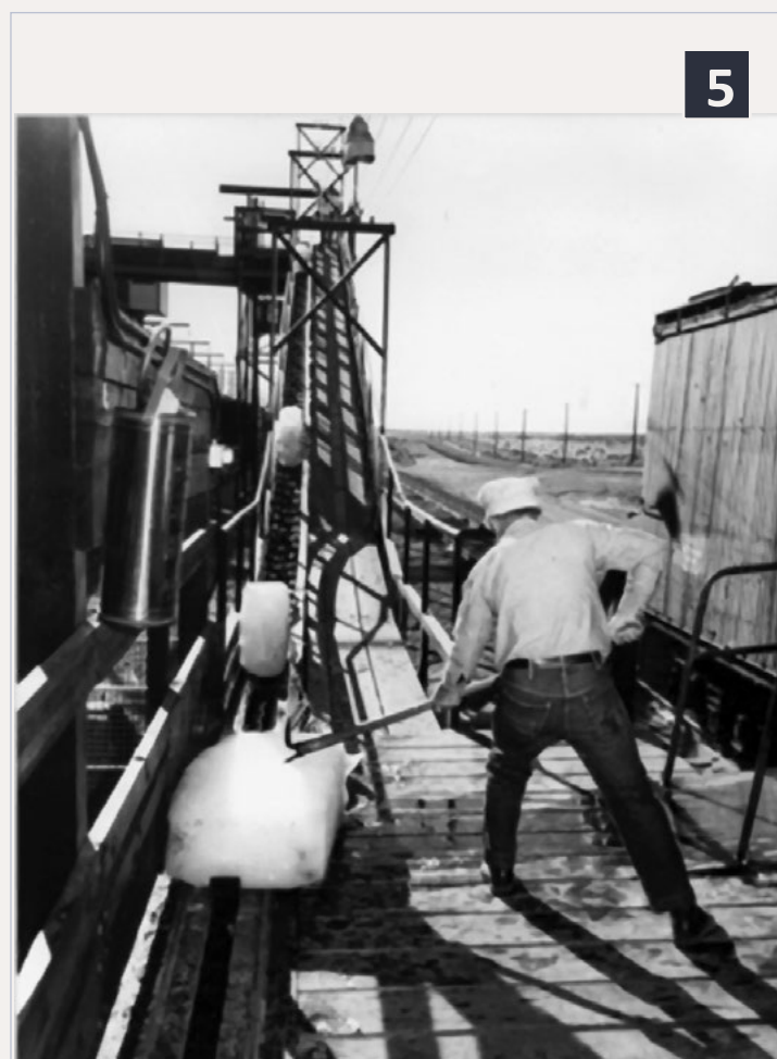
5: A workman uses a pickaroon to manhandle ice out of an ice service car onto the chain which takes it up onto the ice deck at Hinkle, Oregon. – PFE photo, courtesy CSRM.
