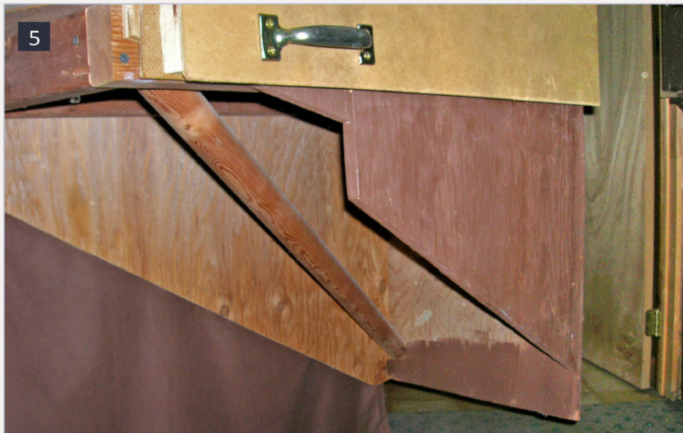
5. Underside of gate.
