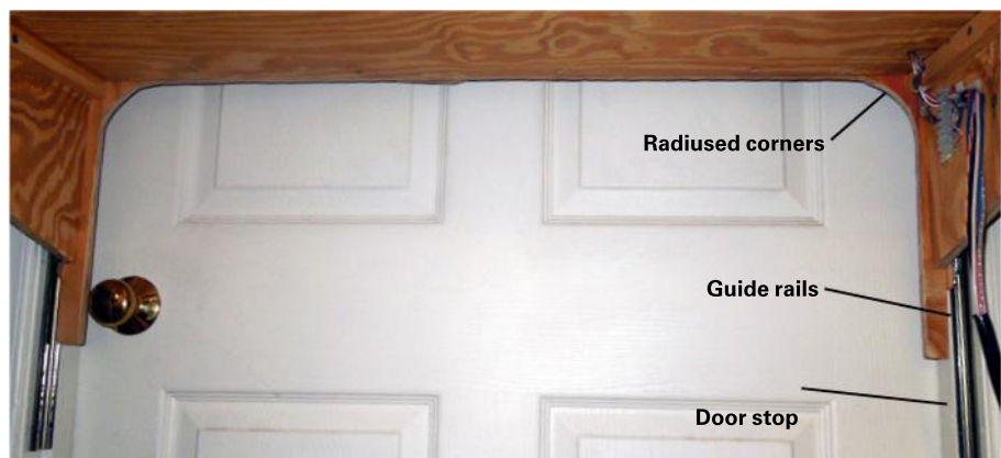
Fig. 3 Radiused corners and drawer glides. James cut the corners of the lift-up section as a curve to reduce cracks. The drawer glides are installed inside the jamb on the non-swing side of the door frame.
